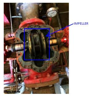
water flows through the center of the pump it passes a rotating impeller. The impeller flows the water through the inlet side of the pump. The impeller discharges the water under increased pressure through the standpipe system.
