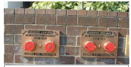
(The left Fire Department Connection in the photo is to cover the lower zone and the right Fire Department Connection is to cover the higher zone.)
