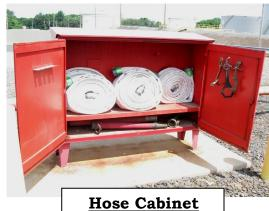
Locking of cabinets shall be permitted in Institutional Group-3. Cabinets containing fire-fighting equipment such as standpipes, fire hoses, fire extinguishers or Fire Department valves shall not be blocked from use or obscured from view. Hose valves are capped with a hose valve cap fastened to the valve with a chain.
