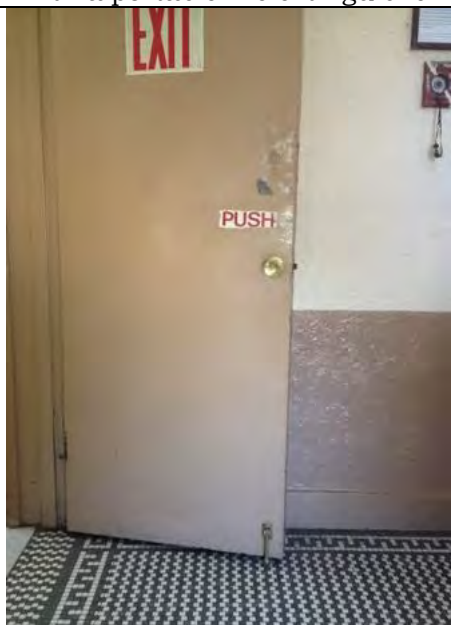
Fire doors illegally propped open with a portable fire extinguisher
