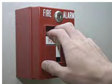
Activating a single action station
