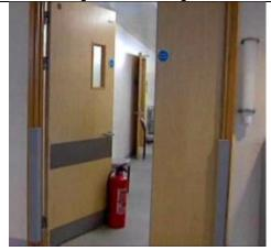
Fire doors propped open using a portable fire extinguisher (illegal)
